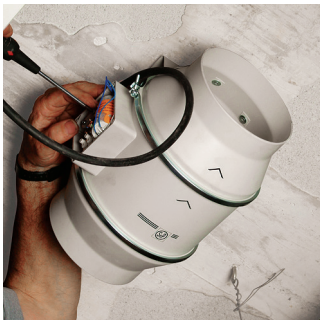
Carry out the wiring connections.
