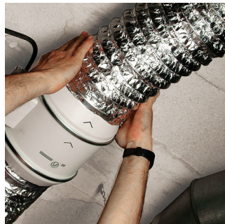
Connect the ducts.
