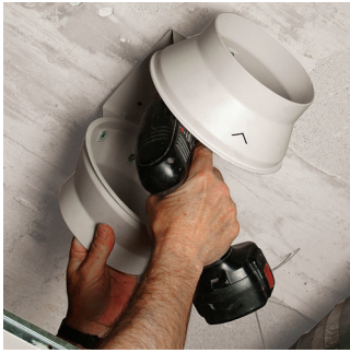
Fix the support bracket.
