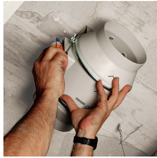
Place the impeller and motor.
